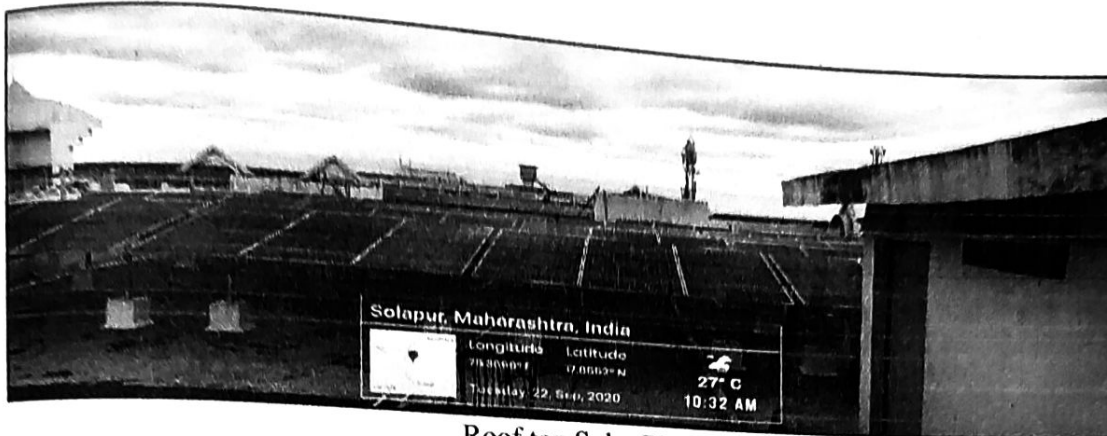
Roof top Solar PV
